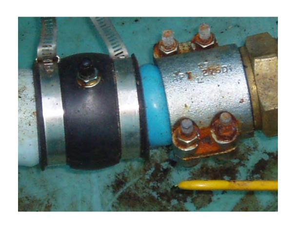
Piping interstitial space is open to the sump (Open systems only, N/A if closed system or not conducting interstitial monitoring)
