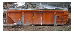
• Sediment tank/filter box: A tank structure constructed from steel drums, modified dumpsters, wood, or other materials filled with sand, gravel or other material to trap and filter slurry water. Portions of the structure after the filter media may be perforated to allow discharge to the surface or have a discharge port to pipe
