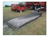
**include:** •Sediment Filter Bag: This device traps sediment while allowing water to flow through the bag. Sediment captured in the bag can be spread on vegetated land following use. It is important to
