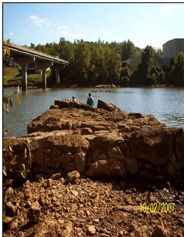
Figure 4. Exposed bridge pilings from an old bridge (from the Catawba Riverkeeper)
