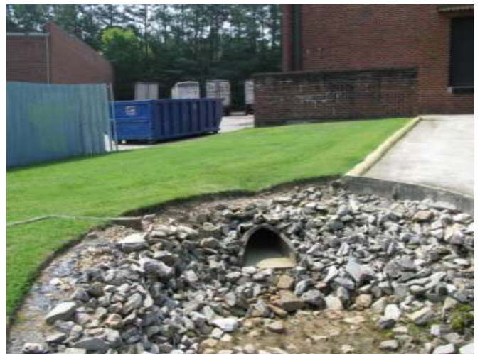
Figure 18: Dumpsters on impervious surfaces draining directly to stream system
