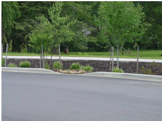
A small curb cut allows stormwater from a parking lot to enter into a bio-retention area bordering the parking lot.
