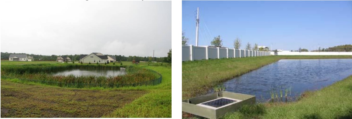
Figure 4.8 Examples of Wet Detention Ponds
