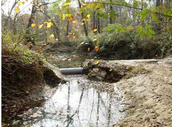
Lexington sewer crossing causing upstream erosion (B-01)
