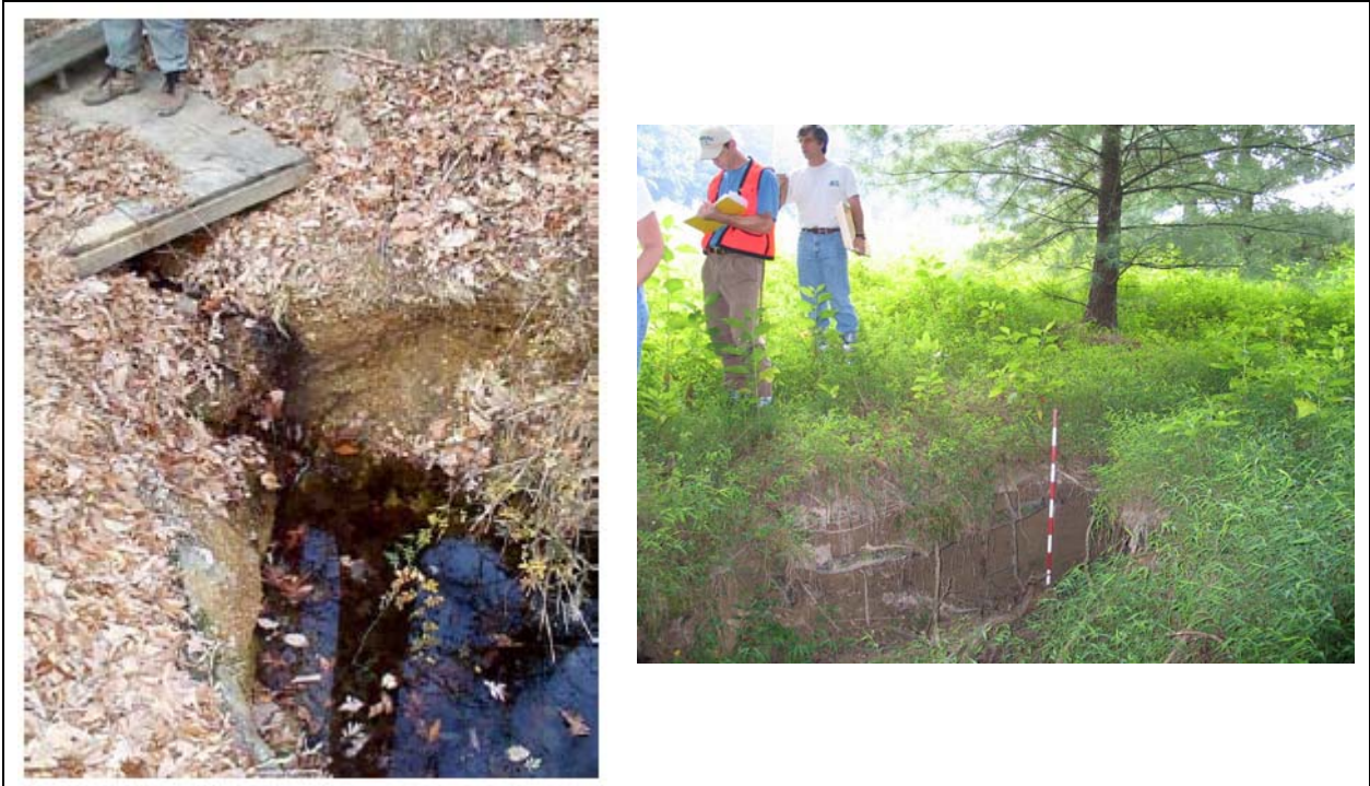
Figure 5. Examples of headcuts (Striped stick is 1.0 m long, painted in decimeters)
