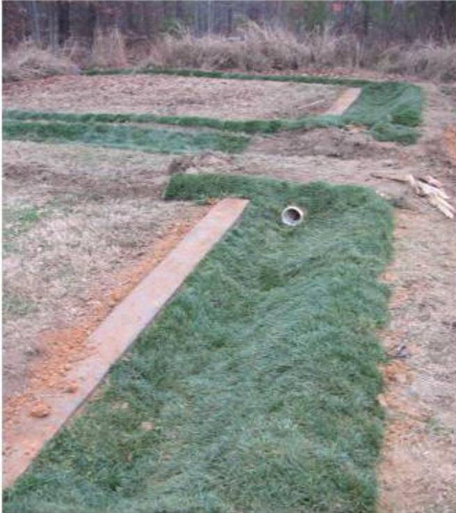
**Figure 8-17:** LS and Blind Swale Post-Construction
