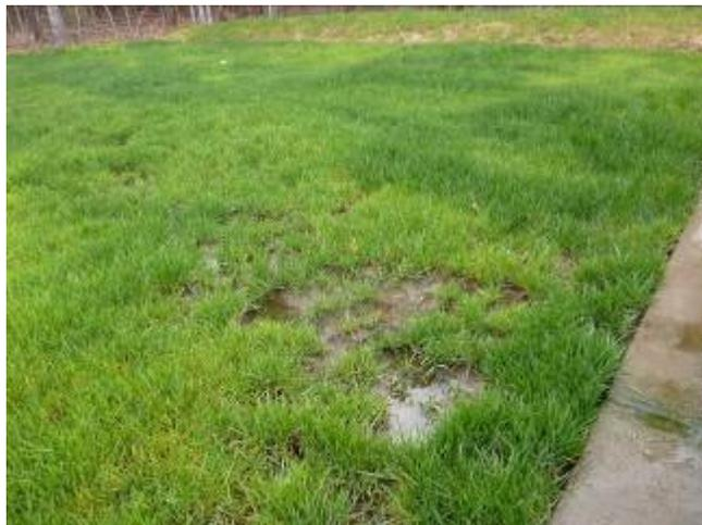
**Figure 8-21:** Erosion in the VFS
