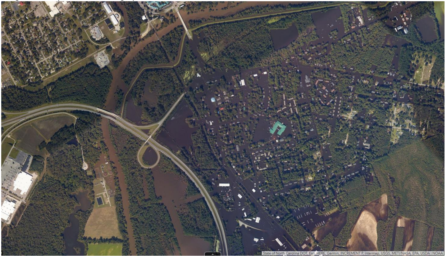
Figure 4. Tar River in Tarboro, Princeville, N.C. 10/13/2017, N.C. 33 & U.S. 258 Intersection Image courtesy NOAA NGS Imagery Services
