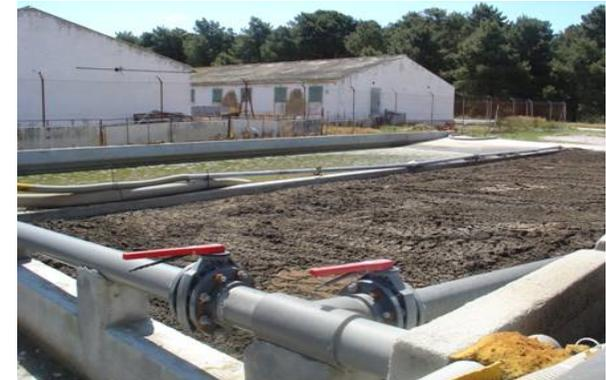
Ammonia recovery from livestock manure using gas-permeable membrane module and concentrator tank (Closed loop system).
