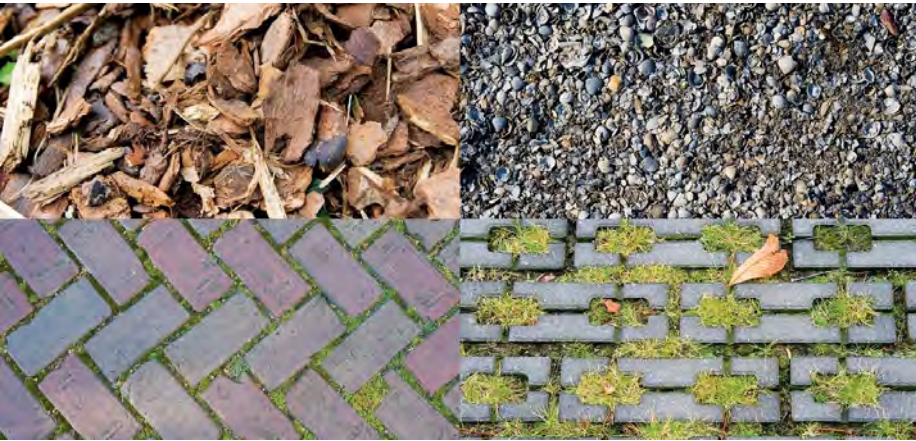
Figure 1: Examples of permeable surfaces (left to right): Woodchips, Gravel, Bricks & Grass-concrete
