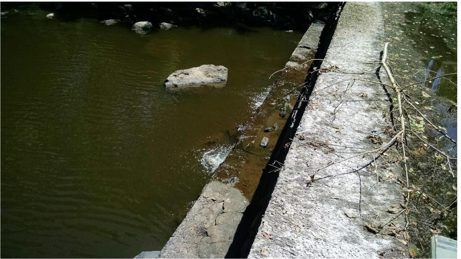
Figure 2. Sluice gates of Hackney Dam, taken 6/13/2016 by ISB staff
