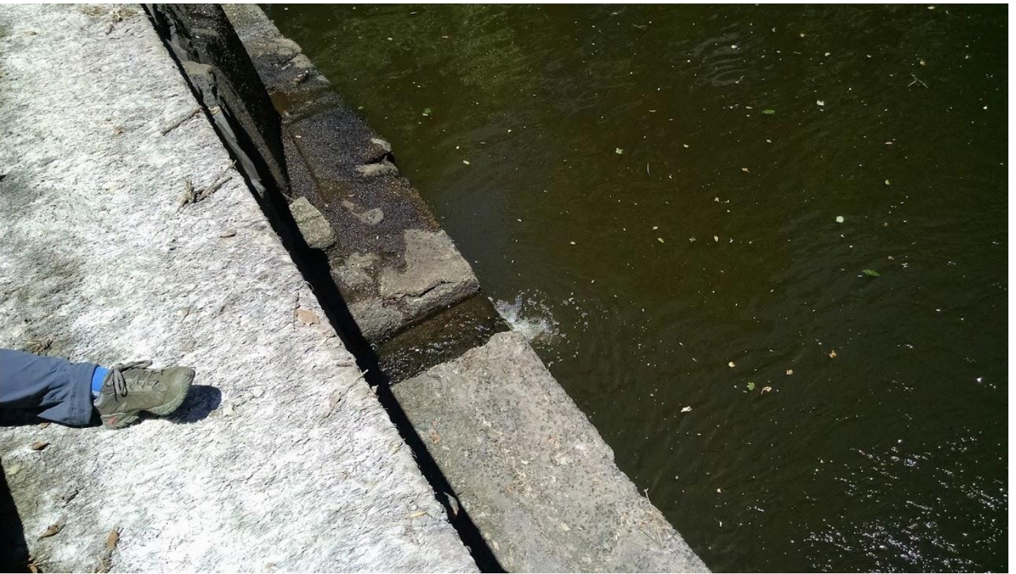
Figure 3. Looking Downstream of Hackney Dam, taken 6/13/2016 by ISB staff
