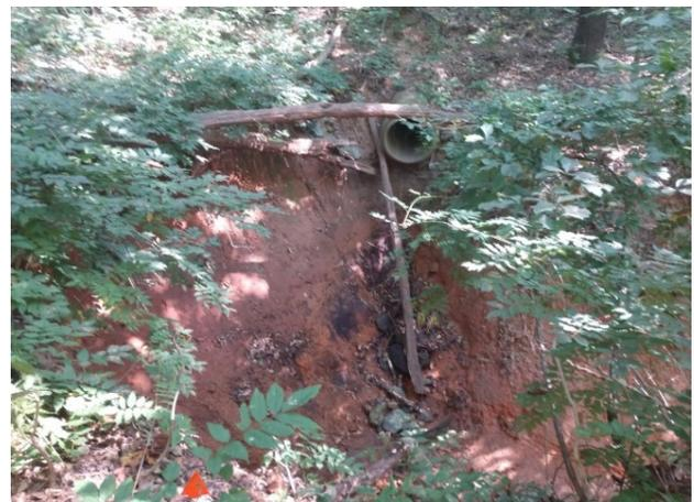
*Figure 47 Erosion plunge pool at stormwater outfall.*
