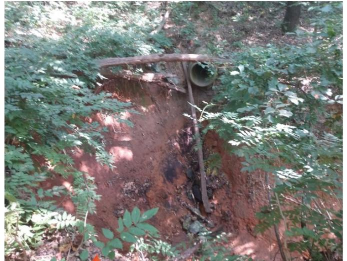
Figure 21 Perched stormwater outlet and 13 feet deep plunge pool below A-B Tech campus
