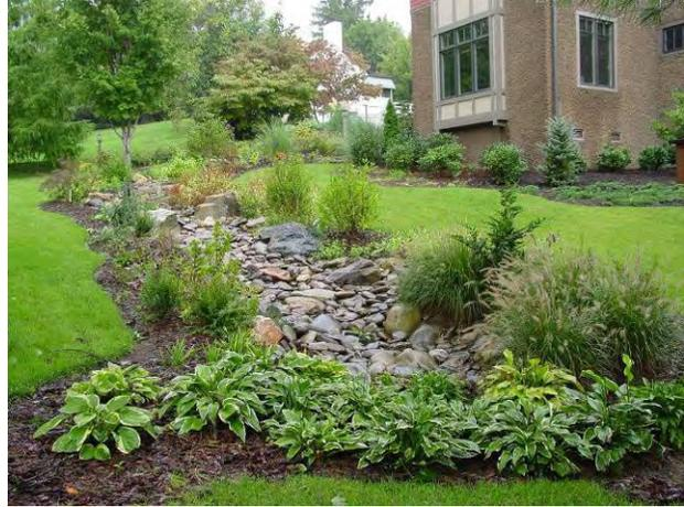
The rough edges of the stones and the interstitial spaces in between slow down runoff and allow it to be absorbed by the ground. Landscape plantings within and surrounding the dry creek bed also slow the water and promote infiltration. The stones and plants can also work together to create natural habitat for birds and small mammals.
