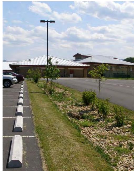
Examples of Bioretention Used in Medians at a Parking Lot
