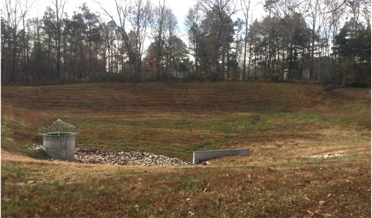
Figure 4-2. Example of a retrofit opportunity in an existing dry pond (SCM Site 00267 located along Keohane Drive in the Mud Creek watershed). The site is likely too small to accommodate a full-sized wetland but water quality could be improved with the proposed retrofit, a pocket wetland.
